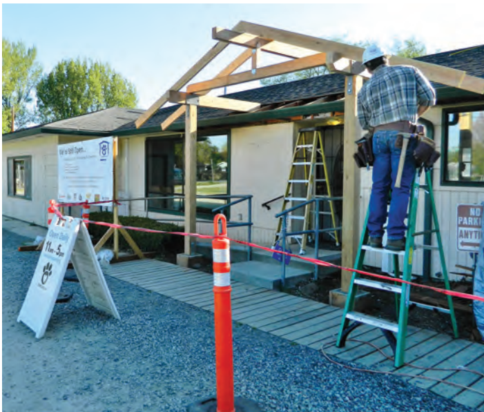
Adroit Construction at work
