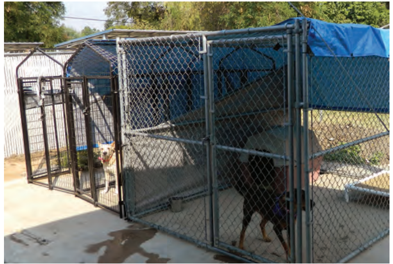
Stray hold kennels will receive a new year-round weatherproof metal roof
